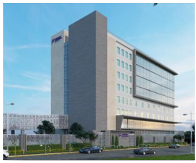
Hospital ChristusMuguerza, Monterrey
