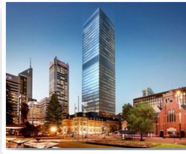
Old Treasure Building, Australia
